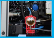
Packaged to work. From day 1. Oil Auto Top Off System, NG/LP Toggle Switch, utilizing modern controls we monitor all engine performance along with power quality - with on screen codes and diagnostic information.
