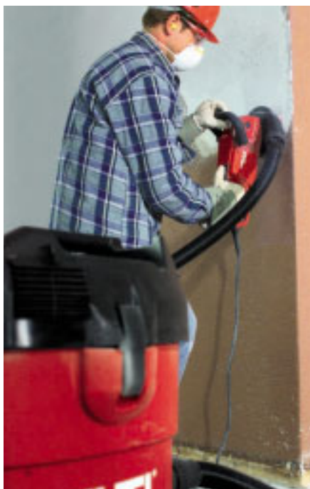
Removal of thin paint coatings on hard cement rendering
